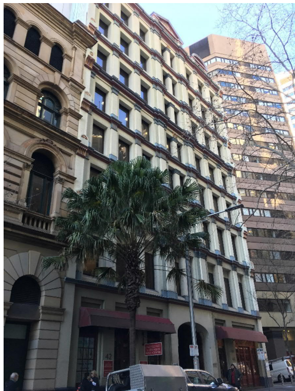
Figure 3.5 View of the former warehouse Gerling House. (Source: GML Heritage, August 2019)
