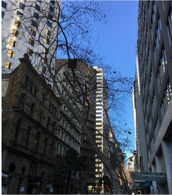
Figure 3.6 View looking south from the corner of Pitt and Underwood Streets. The heritage items are shown opposite (on the left), as is the visual relationship with the subject building (on the right). (Source: GML Heritage, August 2019)
