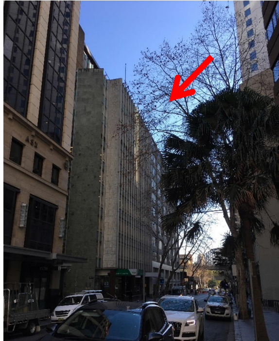
Figure 3.11 View north from the intersection of Bridge and Pitt Streets (in front of 46–50 Pitt Street). The Lend Lease Circular Quay Tower (LLCQ) (under construction) would occupy the same footprint as the former tower at 33-35 Pitt Street (see Figure 3.11) and be visible at this location. The proposed tower on the subject site would be visible against the background of the LLCQ tower. (Source: GML Heritage, August 2019)
