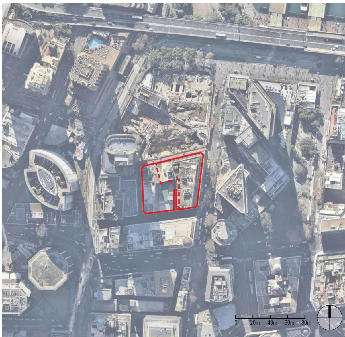
Figure 1.2 Aerial photograph showing the subject site (outlined in red). The dashed line demarcates the building envelope (eastern half), comprising 37–57 Pitt Street and 6–8 Underwood Street. (Source: Google Maps, March 2019)
