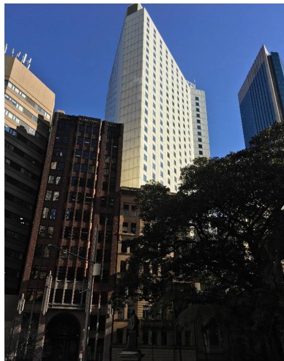
Figure 3.9 View northwest of the heritage items in Macquarie Place, against a backdrop of the Marriott Hotel. The subject site is not visible from this location. Therefore, the proposed development would not affect the heritage significance of these heritage items. (Source: GML Heritage, March 2019)
